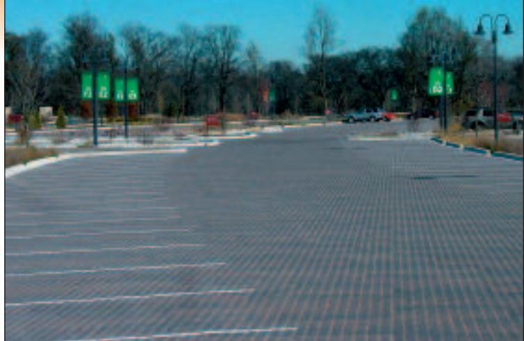
The new parking lot at The Morton Arboretum in Lisle, Ill., proves pervious interlocking pavement is gaining acceptance. The portion of the lot in the bottom-left-hand side of the photo at right is ADA-compliant; the top-right portion is not.
